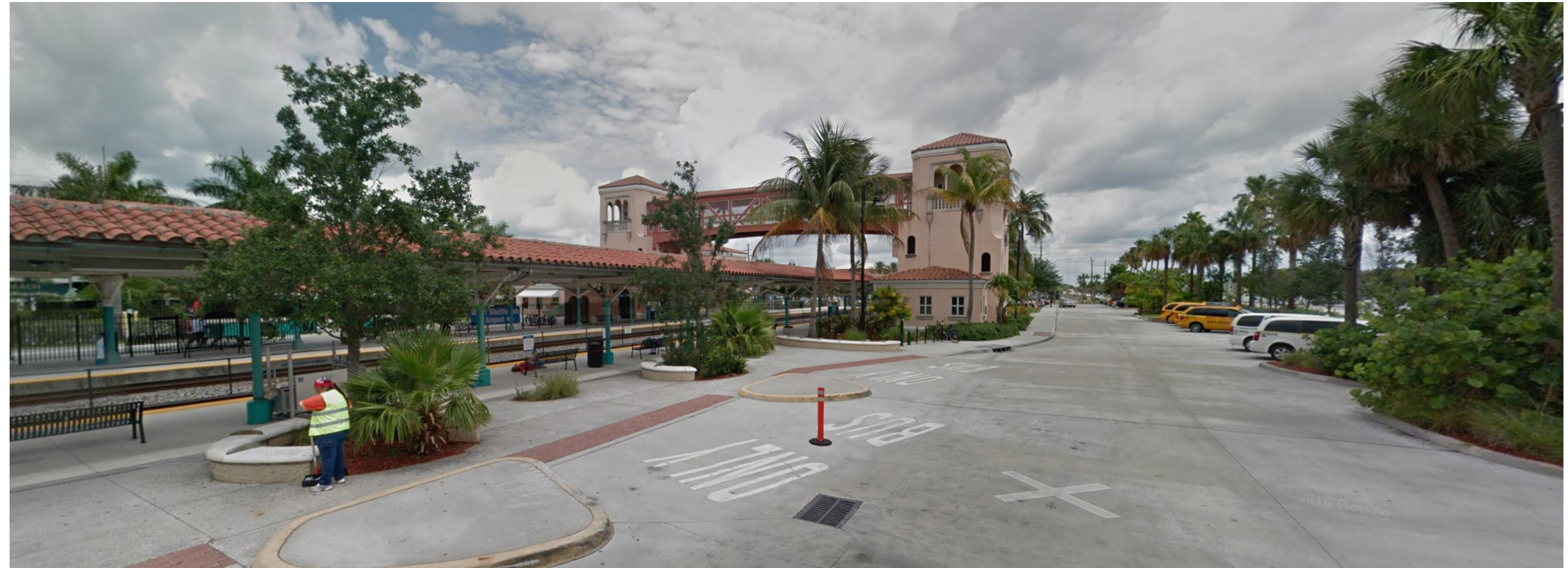
West Palm Beach Tri-Rail Station, WPB, FL
